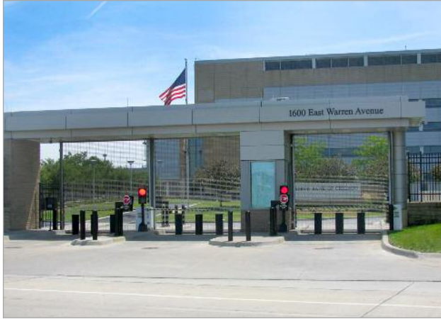
Ideal Contracting, Inc., the general contractor for work at the Detroit Branch entrance, was among the top MBEs awarded work with the Chicago Fed in 2014.
